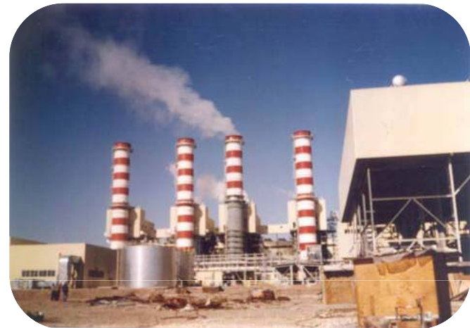
Ghom, Combined cycle power plant
